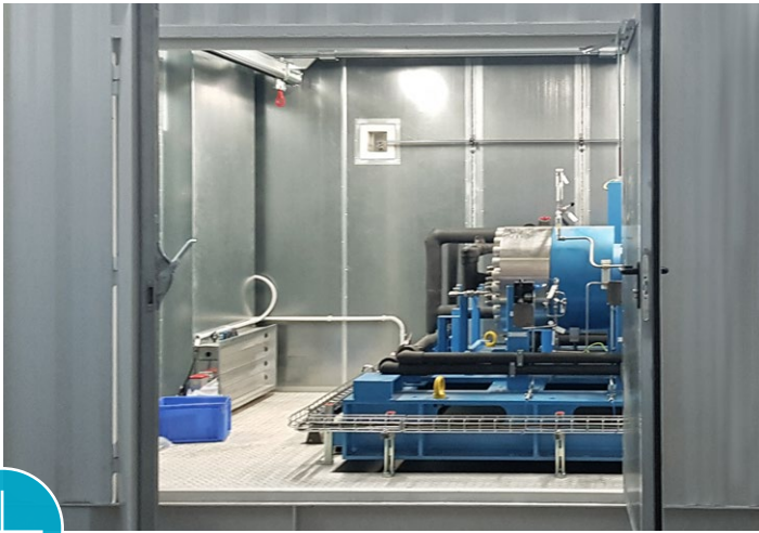
Diaphragm compressor for reliable refuelling of the bus fleet
